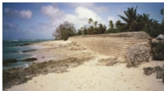
Fig. 3. Typical seawall used to prevent erosion. Note, sand has been removed in front of seawall.
